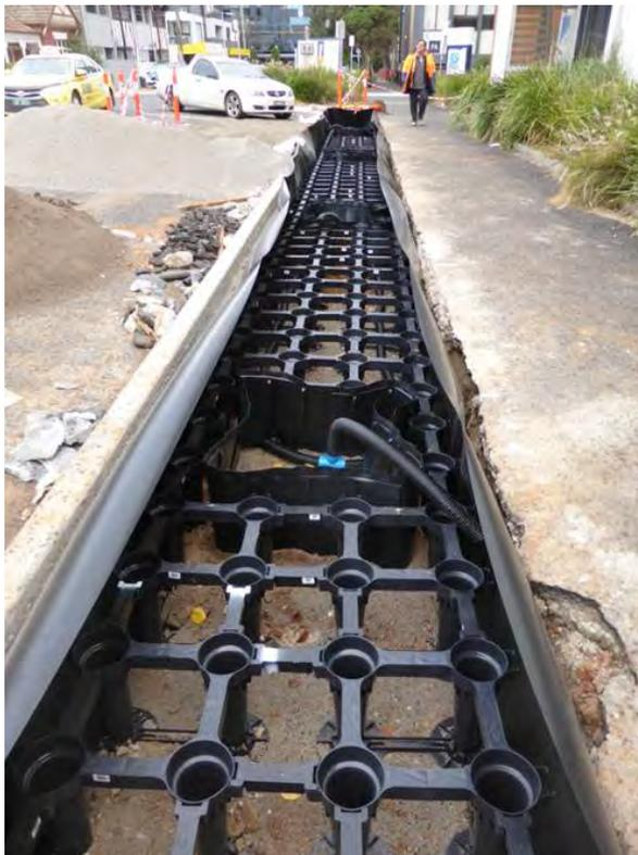
Figure 46: Trench of soil cells prior to the addition of uncompacted soil (Photo Source: Steve Watt, Stonnington City Council)
