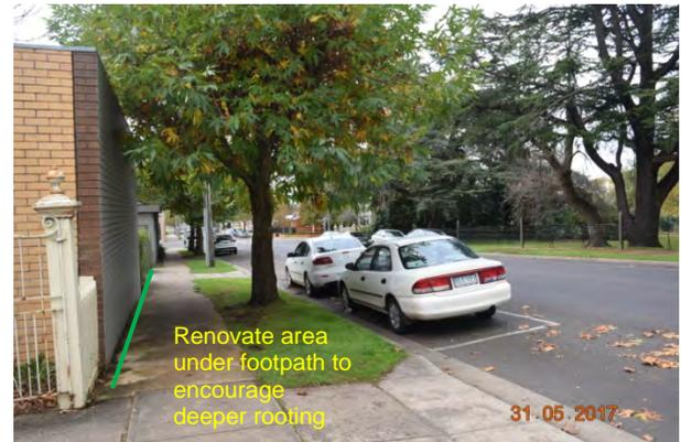
Figure 35: Option 1 recommended measures - install root barrier (green) and renovate below ground space under footpath
