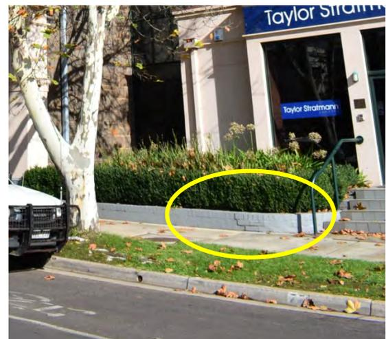
Figure 22: Minor cracking of retaining walls
