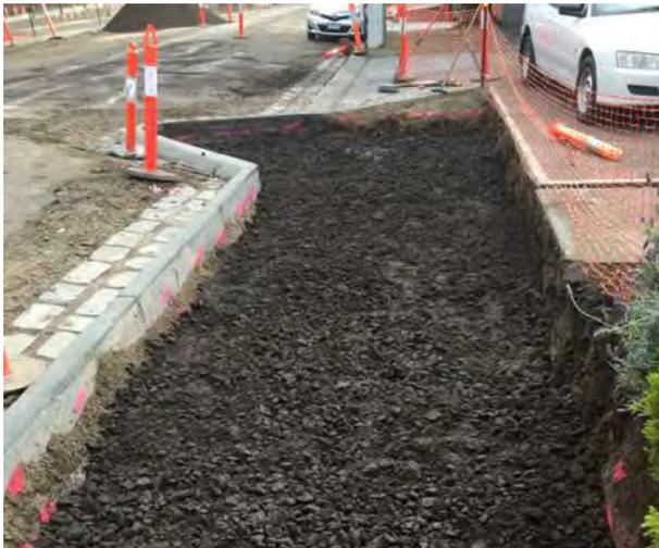
Figure 44: Structural soil installed under footpath for root growth (Photo Source: Steve Watt, Stonnington City Council)
