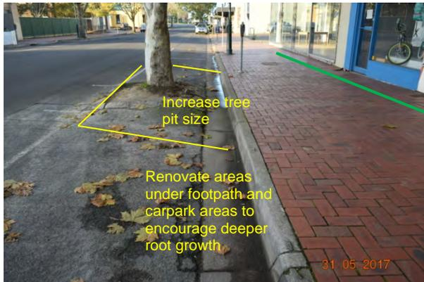
Figure 34: Option 1 recommended measures – increase tree pit size (yellow), install root barrier (green) and renovate below ground space under pavement
