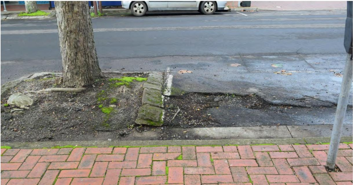
Figure 16: Asphalt damage adjacent to the small tree cut out
