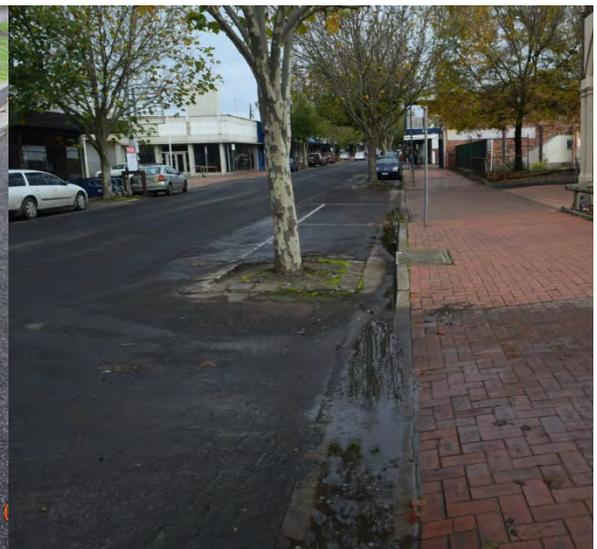
Figure 18: Kerb and channel not functioning as designed resulting in water ponding
