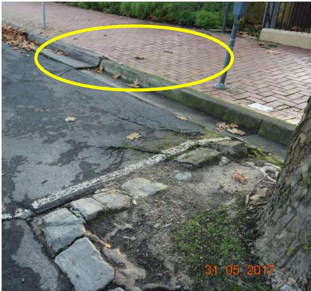
Figure 19: Footpath lifting and asphalt damage presumably in response to root growth
