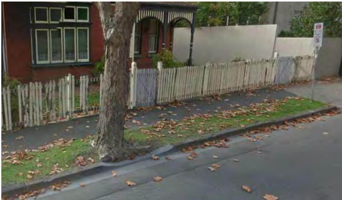
Figure 41: Modified kerb reinstatement method to allow space for buttressing trees roots and maintain effective road drainage (Photo Source: Steve Watt, Stonnington City Council)
