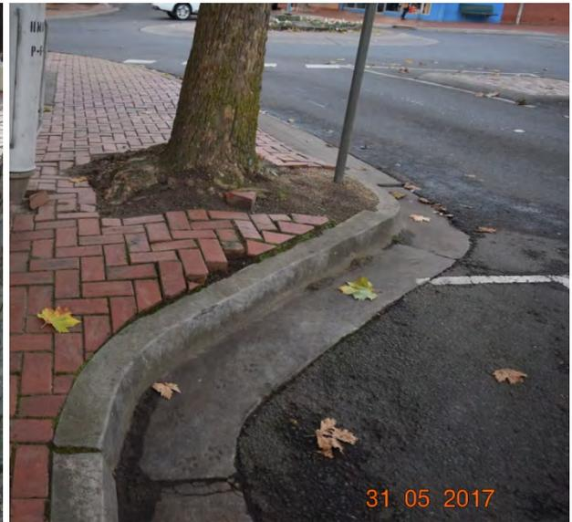
Figure 20: Brick pavement is prone to movement, creating uneven surfaces
